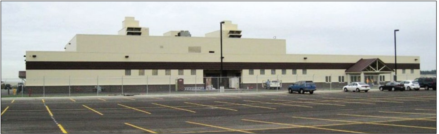
The F22 LO Maintenance Facility design-build project at Joint Base Elmendorf-Richardson was the first facility built to support the F-22 Wing.
